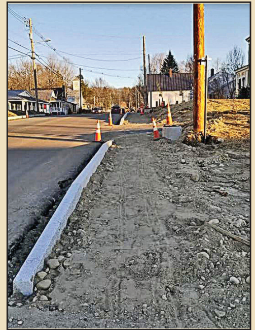
Installing granite curbing.
